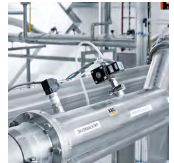
Air intake ports for secondary air
