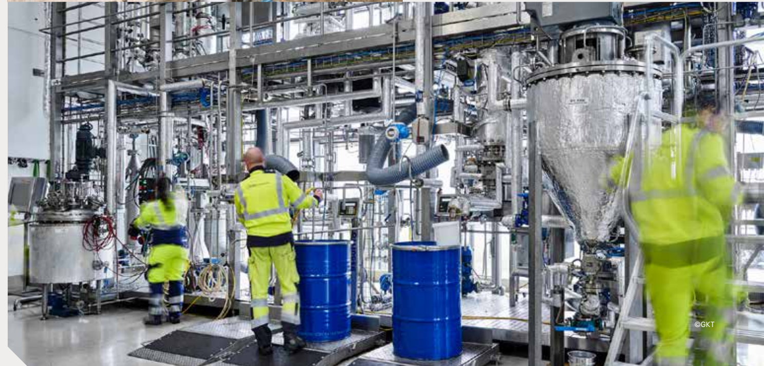
➤ GKT technical center in Gloggnitz, Austria
